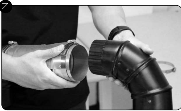
7 Fit 3" 90° Elbow inside 3" Ducting Tee. Ensure that the 90° Elbow is facing downward, and the branching vent of the Ducting Tee is facing to the left.
